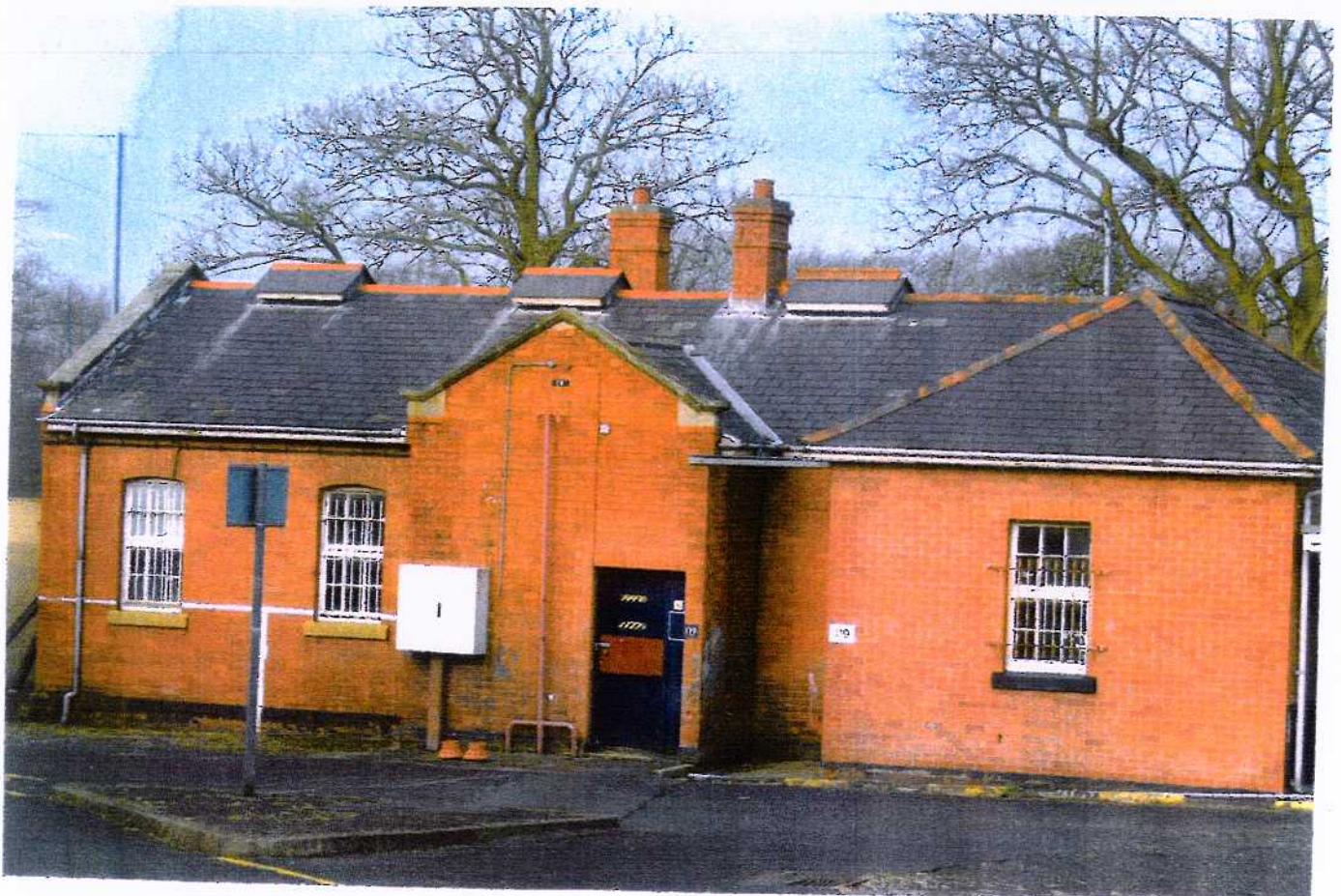
This little red brick building is on the 1904 map, but its use is not known. It was a 'cold store' on the 1948/52 plan and is numbered 119 on the EHS plan. (A.J. Malley)
