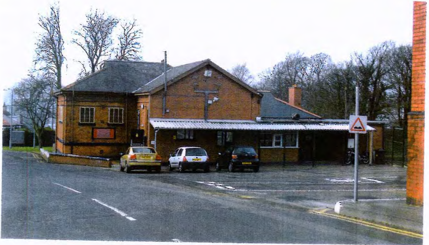
This image is of the former guard house for the barracks and in 1948/52 was a store house. It appears to have been rebuilt after the Second World War and originally had a basement which held the barrels of rum for the sailors daily ration. It may well still be there underneath the present guard house. (No.102)
