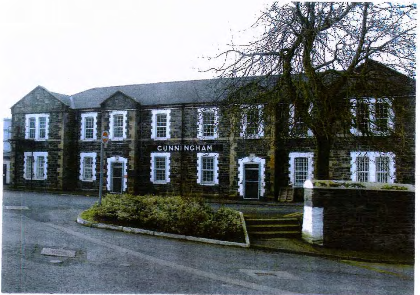
This stone built block was erected after 1875 as part of a barracks extension. It was named as 'Cunningham Block' on the 1948/52 plan and is numbered as 4 on the EHS plan. (A.J.Malley)
