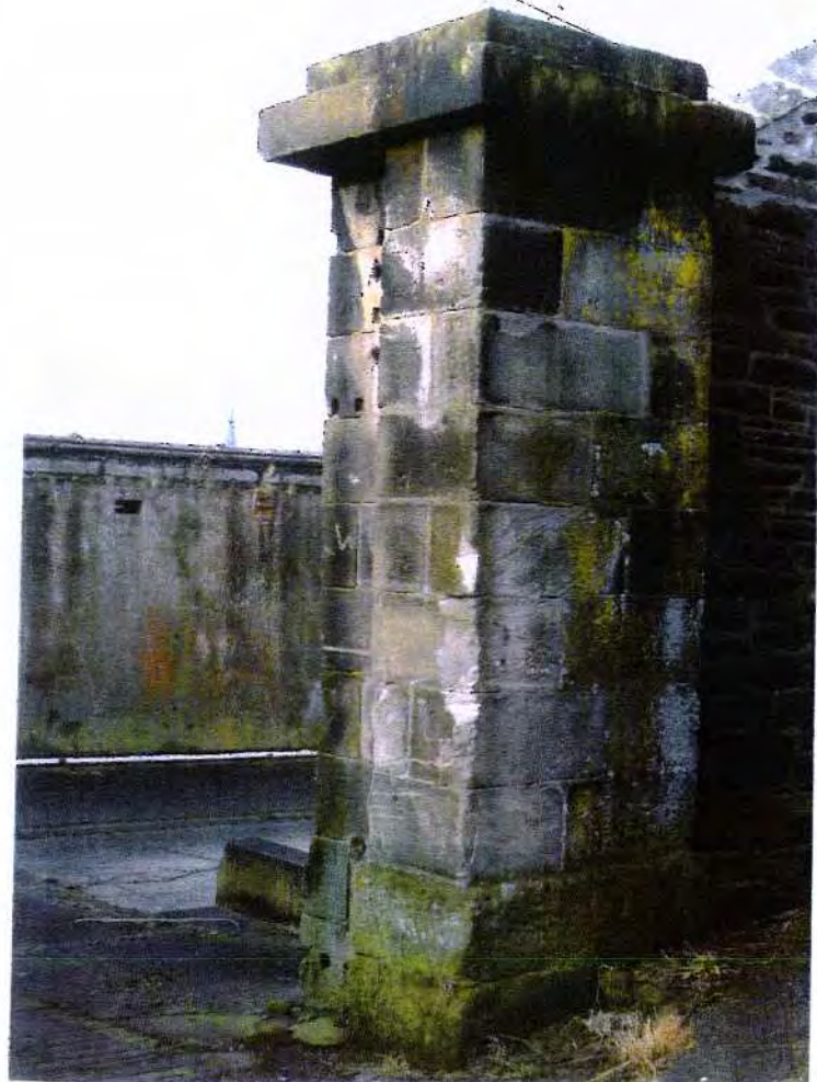
Stone gate pillar of old oval yard erected in 1841 and was used as a fuel store and Engineer's yard. The 1948/52 plan shows such uses as 'Chief Engineer's yard, store and coal pound'. The walls etc will be Scheduled by EHS. (A.J.Malley)
