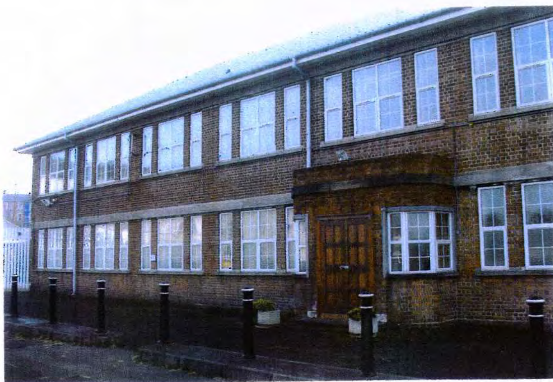
Part of 8 th Brigade HQ building erected after 1949 and houses original foundation tablet etc. This building was named 'XC H.Q' on the 1948/52 plan and is numbered 25 on the EHS plan. (A.J.Malley)
