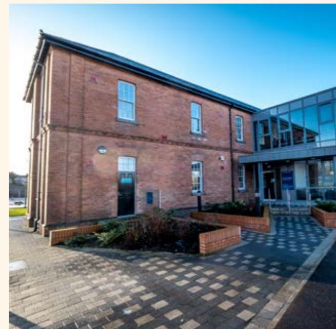
Building 104 | Small-medium enterprises
